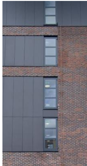
White Mortar Recessed Brickwork
